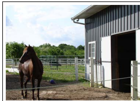
Clean water diversions like rain gutters help reduce mud and keep clean water clean.
